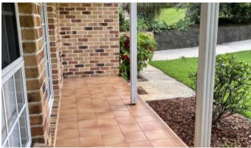
Unit 1, 2 Cerreto Cct, Wollongbar
